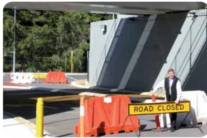
Bill recently inspected the Karrakatta underpass.
